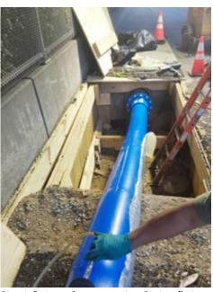
Liner inflation and pressure testing after installation
