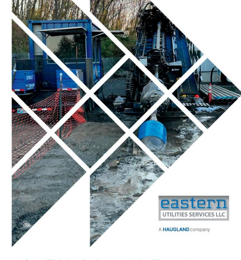
Eastern Utilities Services LLC provides horizontal directional drilling, auger boring, microtunneling and other services in connection with trenchless installation. Our fleet of specialty drilling equipment is capable of tackling any size project with pullback up to 1 million pounds.
