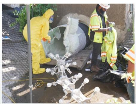
The light chain was pushed and pulled in a timed sequence to cure the inflated liner to the host pipe
