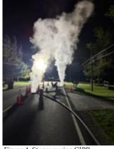
Figure 4. Steam curing CIPP
