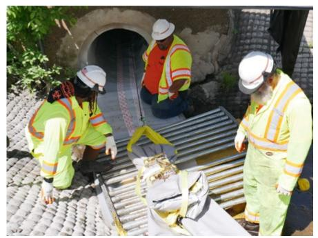
The UV CIPP liner was dragged into place inside the drainpipe using rollers and a winch cable
