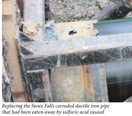
Replacing the Sioux Falls corroded ductile iron pipe that had been eaten away by sulfuric acid caused by sewage, the HDPE pipe is inserted into the destroyed pipe using the CompressionFit method from Murphy Pipeline
