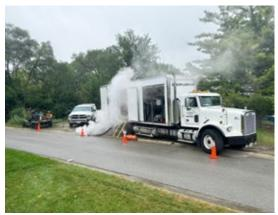
Figure 3. Main sewer CIPP lining
