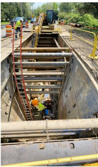
Safely engineered shoring was important considering the depth of the jacking pit
