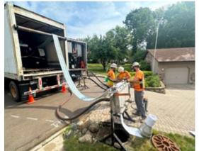
Figure 5. CIPP Liner Installation
