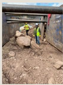
BEFORE: A worker stands next to boulders retreived during excavation of the launch pit
