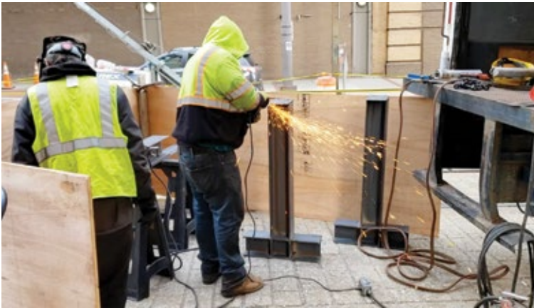
Figure 11: Construction of the steel tunnel system
