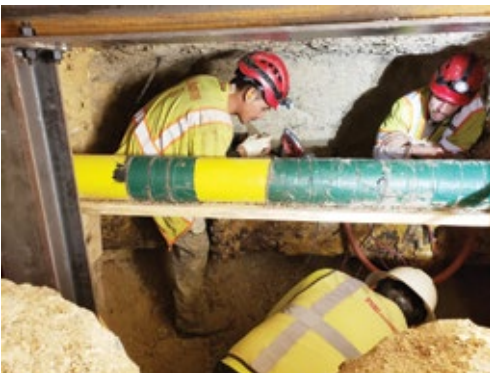
Figure 12: When tunneling towards the valve, a large gas line was encountered
