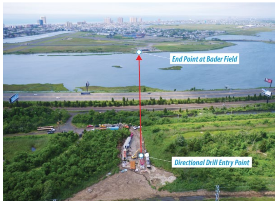
The HDD path for the HDPE pipe under the Atlantic City Beach Thorofare waterway. (PHOTO COURTESY OF ACUA)
