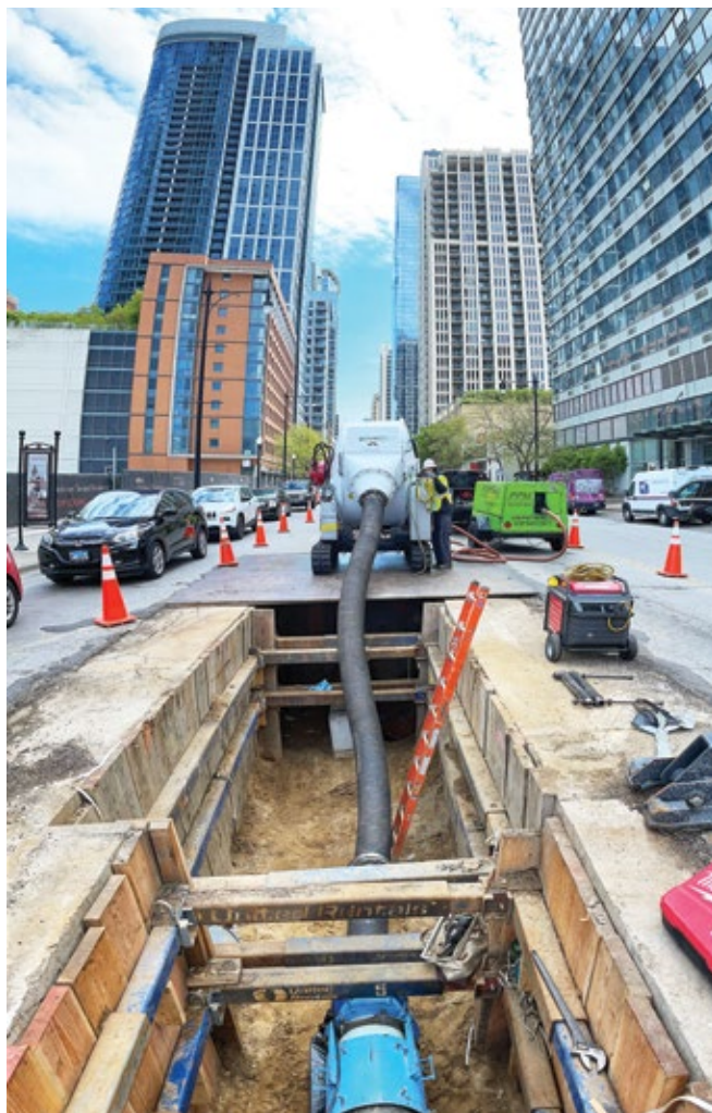
Lining project in Chicago for 20-inch cast iron pipe dated 1861
