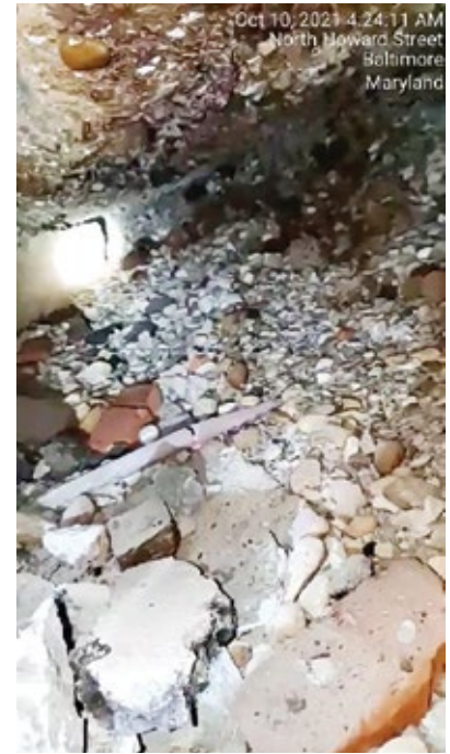
Figure 7: One of the largest voids discovered under the light rail slab
