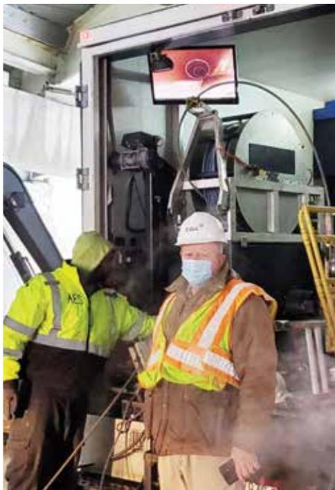
Figure 6. CCTV inspection of pipe in vicinity of the leak required installation of two entry ports
