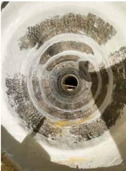
Figure 9. Completed CFR of the 48-inch pipe
