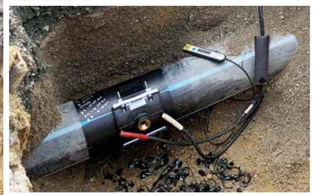
Typical Electrofusion Joint
