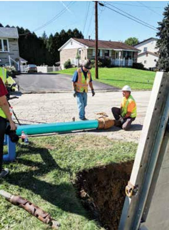
Static pipe bursters allows for the use of a variety of product pipes. Penn Township has been using Certa-Flo® PVC pipe on numerous bursting projects
