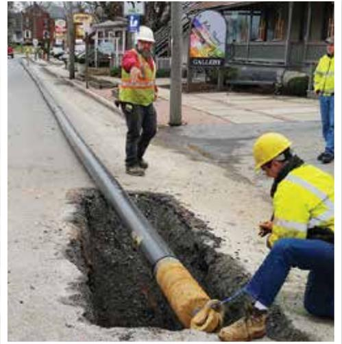
*HDD was used to install new potable water pipeline for Intercourse, PA. Nearly 10 miles of HDPE pipe installed*
