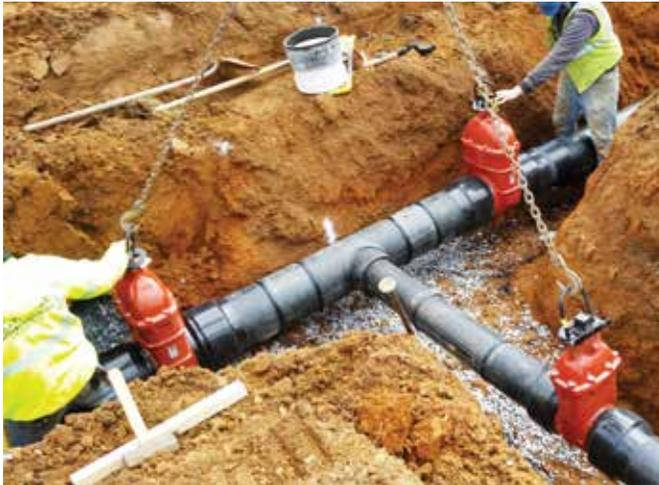
Shut-off valves and fire hydrants were heat fused into the HDPE pipeline to further ensure a leak-free, closed loop system
