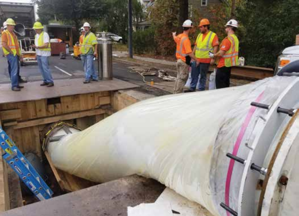
Liner entering host pipe after going through inversion cone
