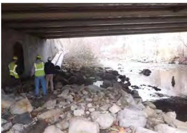
Figure 7 – Bypass Piping Crossing Under Howard Street Bridge
