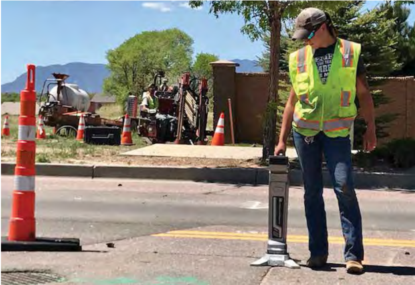
Mag 6 is a versatile and easy to use walkover HDD locating system
