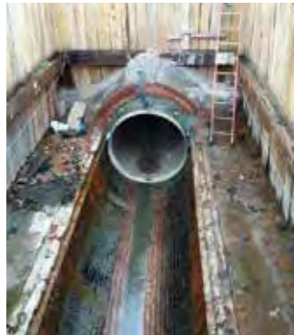
Figure 12 – Sliplining Pipe After Annular Space Grouting
