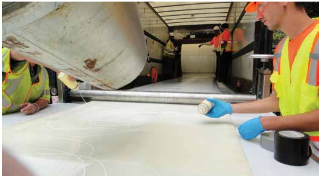
Liner wet out involves mixing two-part chemicals
