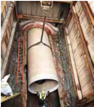
Figure 11 – Sliplining Pipe Placement
