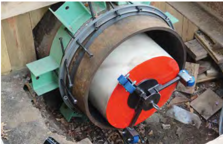
Custom pig fabricated to remove stranded grit
