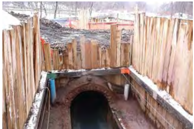
Figure 9 – Trench Shoring and Protection
