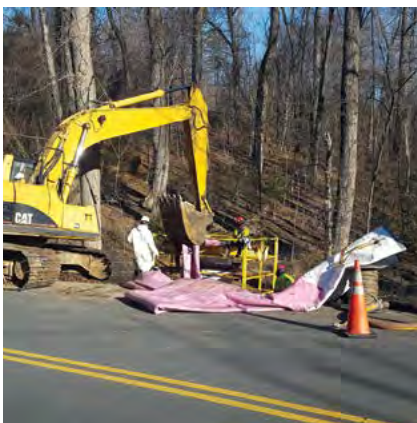
Find and Fix has accelerated the pace of CIPP lining throughout the City
