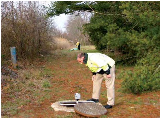
It is not uncommon to inspect over 10,000 feet in a day with a two person crew
