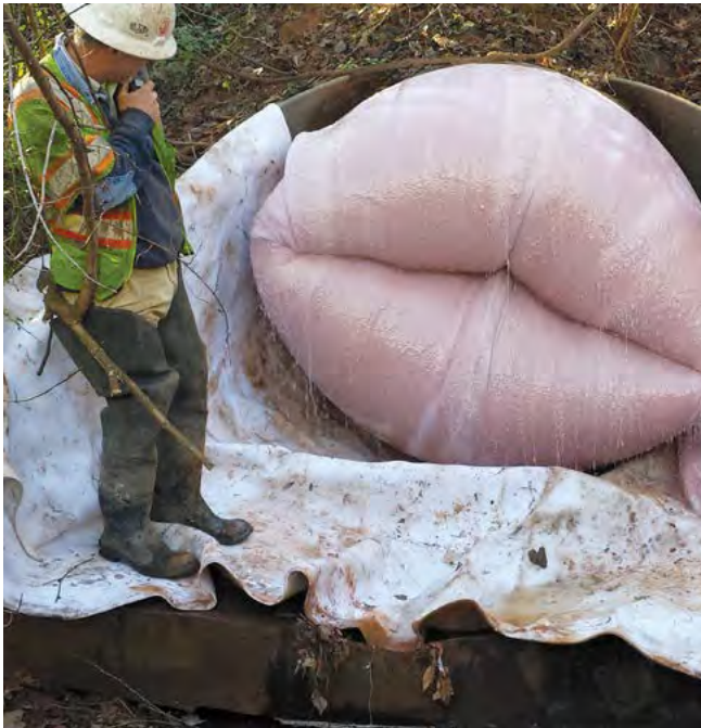
60-inch CMP CIPP. Integrated city-wide storm and sanitary sewer rehab program has streamlined comprehensive rehabilitation of both assets
