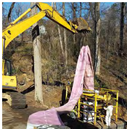
Find and Fix has accelerated the pace of CIPP lining throughout the City
