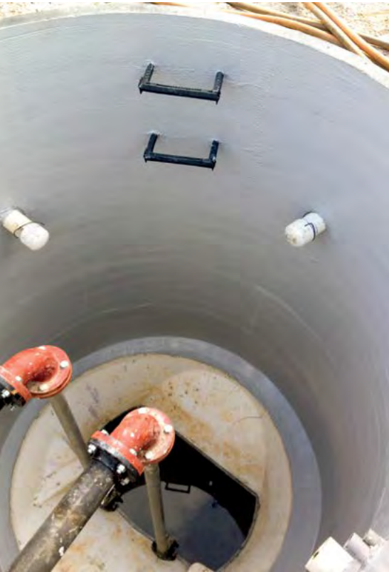
A fiberglass cured-in-place liner can be installed to protect and strengthen any host structure
