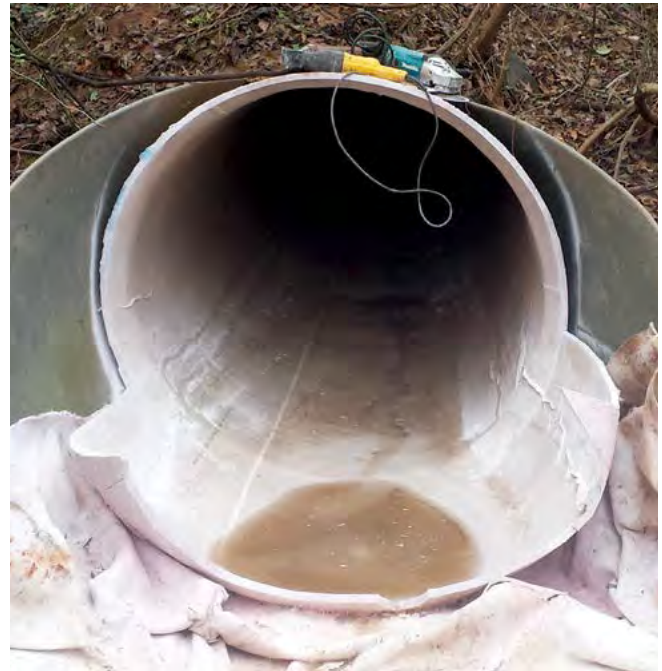
60-inch CMP CIPP. Integrated city-wide storm and sanitary sewer rehab program has streamlined comprehensive rehabilitation of both assets
