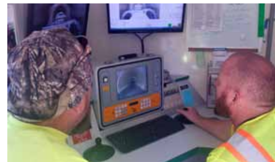
CCTV inspection of laterals during construction
