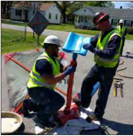
Lateral CIPP installed in bladder system, assembly placed in manhole
