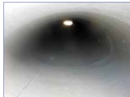
The new culverts are smooth, seamless, watertight, and structurally stronger than the old CMP, with longer projected service life
