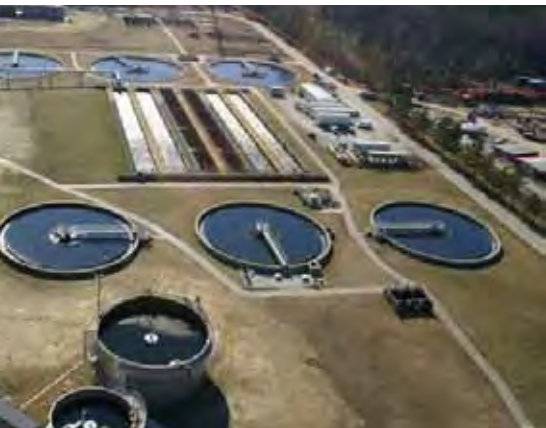
HRSD operates 13 treatment plants
