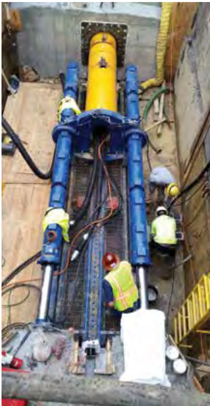
MTBM launch @ College Drive Waterline Project
