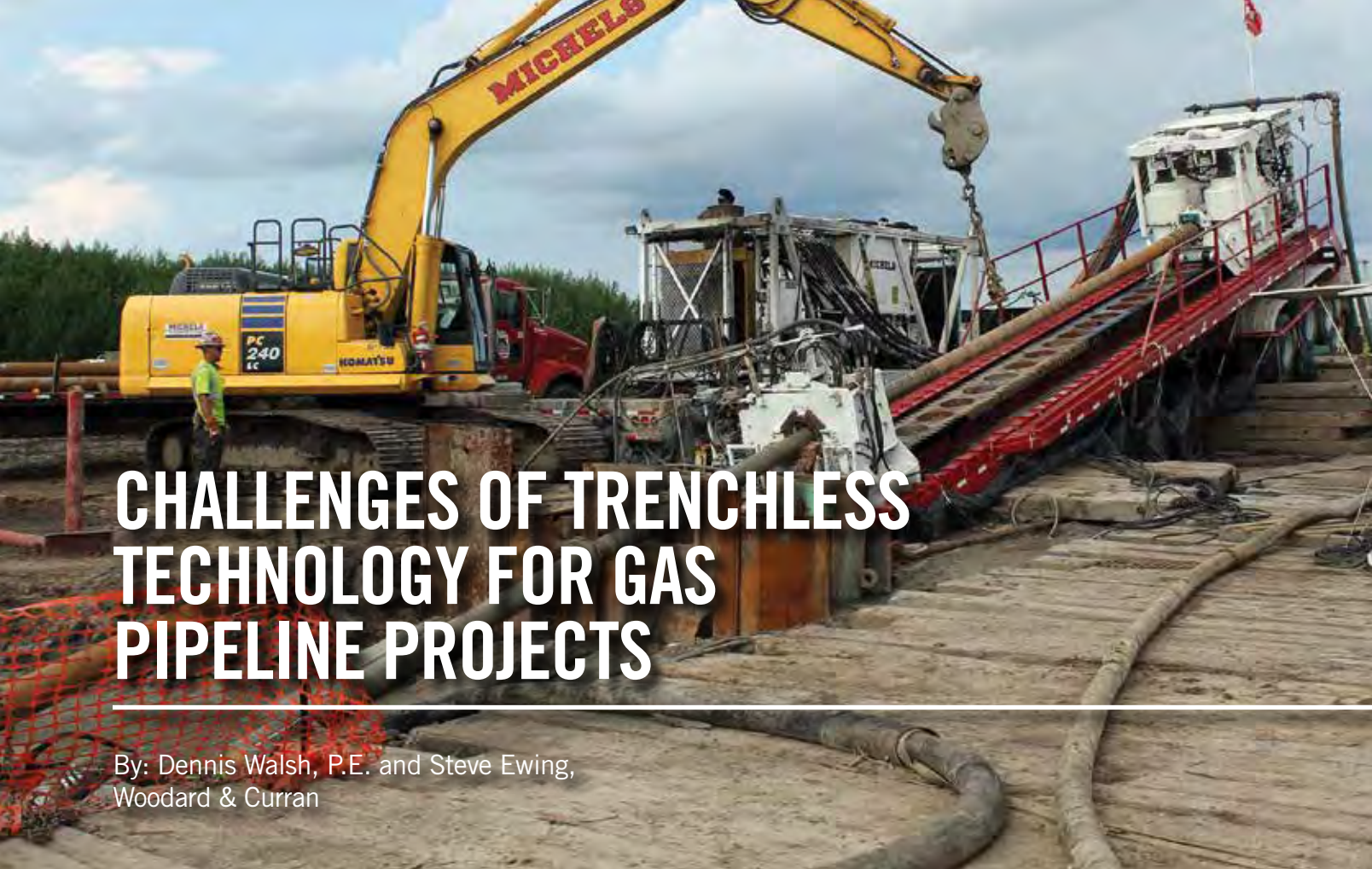
HDD Drill Rig with Control Cab and Mud Pumping Operation
