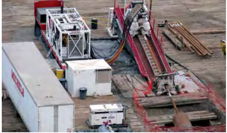
Overview of Typical HDD Drilling Operation
