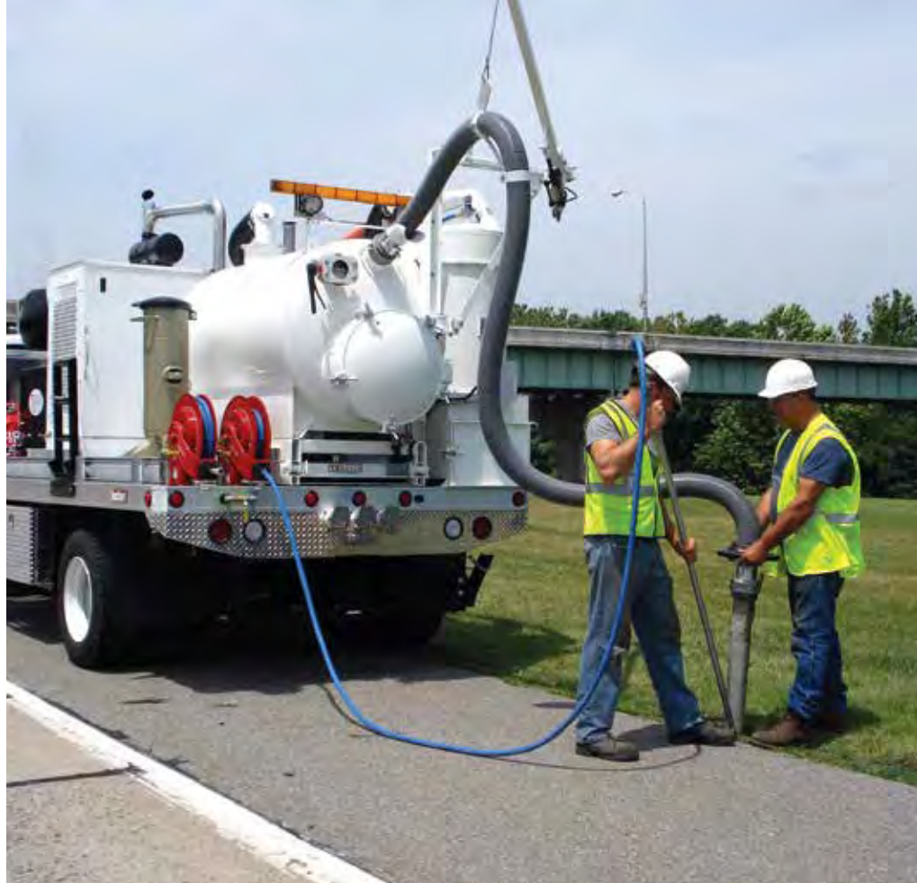
Vacuum excavation rig at work with lighter, more versatile, configuration
