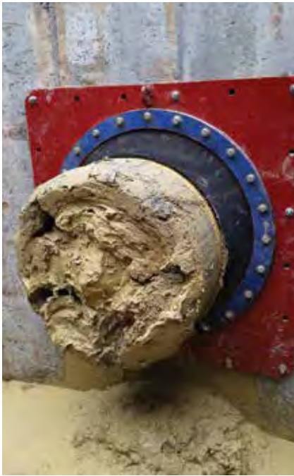
MTBM hole out in wet sand & clay @ College Drive Waterline
