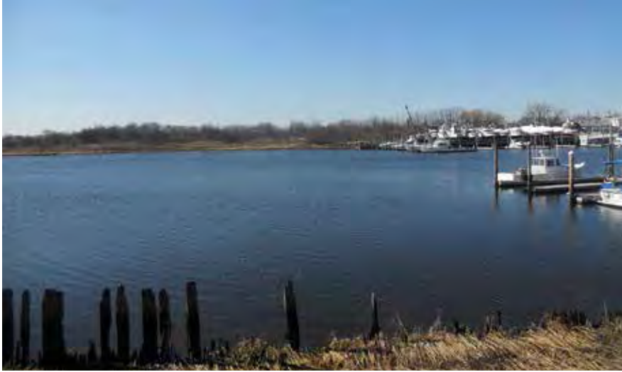
Water Crossing Completed Using HDD
