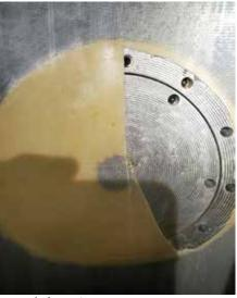
Liner was cut away, plug removed and 20-inch lateral restored after curing
