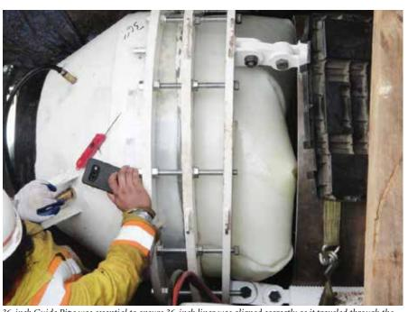
36-inch Guide Pipe was essential to ensure 36-inch liner was aligned correctly as it traveled through the 30-inch segment
