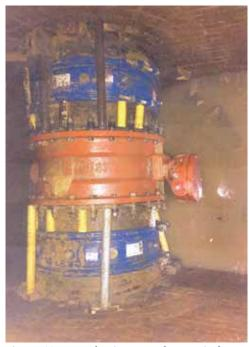
Figure 4. Temporary bracing was used to restrain the new 36-inch butterfly valve while the repair was underway
