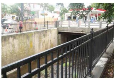
Pipe configuration of "The Mess" was built in 1971 when the Rahway River in South Orange NJ was encased in a concrete channel and the bridge widened
