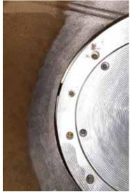
Design engineered prefabricated metal plug installed to cover a 20-inch lateral and provide bearing surface for liner inversion
