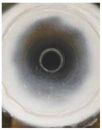
Application of high-strength heated epoxy spray to reinforce and seal leading 36x30-inch reducer was a breakthrough technical accomplishment
