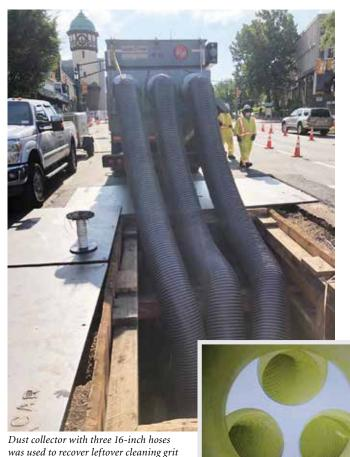
Cleaning began immediately on Monday, and, as with the use of curtain grouting, technical advancements first used during the cleaning phase in the world record 42-inch CIPL the previous year were an essential element in getting "The Mess" ready for lining. The dust collectors and 16-inch inlet hose configuration was used again and generated sufficient airflow to remove any grit leftover from the sandblast cleaning.
