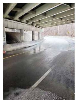
Figure 3. Water main breach was flowing onto the South Bound offramp to I-83, creating hazardous conditions
