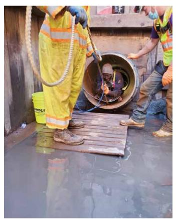
Confined space entry with extensive safety precautions was necessary for several preparatory steps prior to lining
