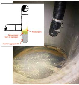
Stack was backfilled, then covered with mastic epoxy to form a 90-degree elbow from the 36x36-inch Tee
