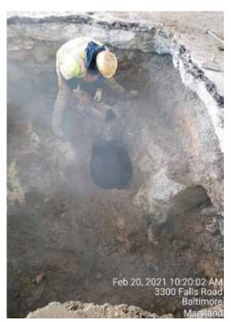
Figure 5. A two-foot hole was cut into the water main to inspect for further damage
