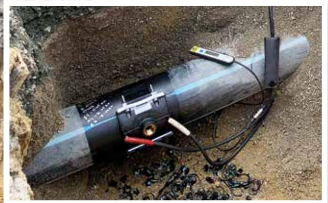
Typical Electrofusion Joint
